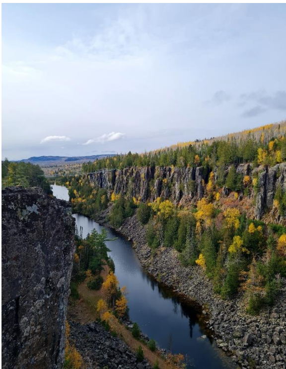
Figure 3: Eagle Canyon Suspension Bridge
